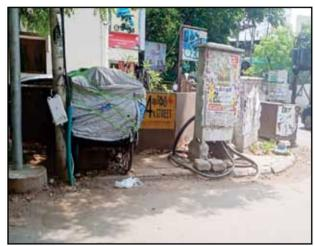
Electric cables outside found lying loose in the street corner of transformer are
