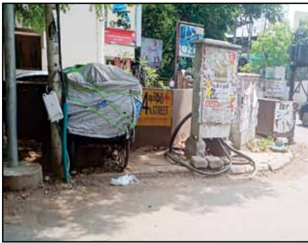
Electric cables outside found lying loose in the transformer are the street corner of
