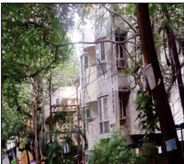
In VP Colony, North Street of Ayanavaram, broken
